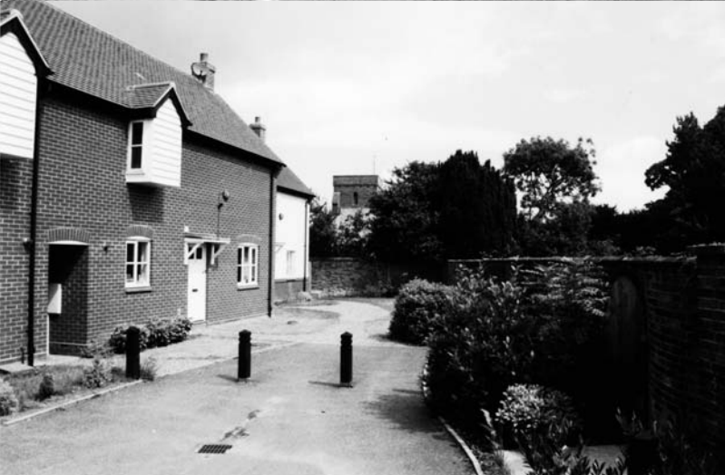
4. This recent development by the Rural Housing Trust has an attractive relationship with the crinkle-crankle wall associated with Bradfield Place. The mature planting of the former vicarage and the churchyard are also important features in this view.
