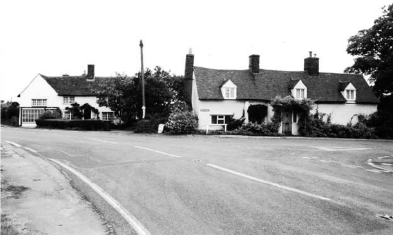
3. Acacia House and Milestones Cottage, with the listed 19 th century milestone between. These listed cottages define the northern edge of the road junction, though the area of tarmac is now rather overwhelming.
