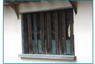
Early mullion window originally unglazed
