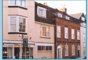
Various historic window styles, Harwich
