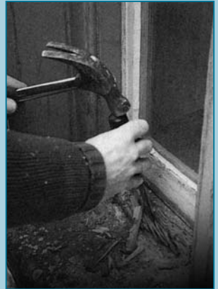
Repair to wooden window frame
