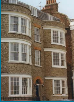
Impressive three storey bay windows in Grade II* Listed Building, Harwich
